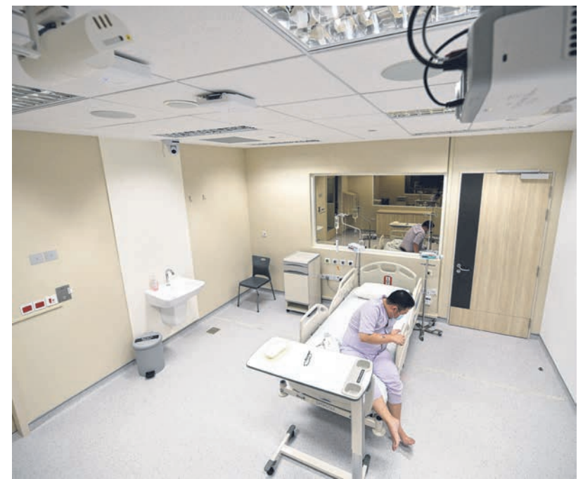
As a patient leaves the bed, thermal cameras installed in the patient's room will send an alarm to the nurses' station. There are plans to deploy the system in all single-bed and isolation rooms at TTSH by the year end. ST PHOTO: NG SOR LUAN
