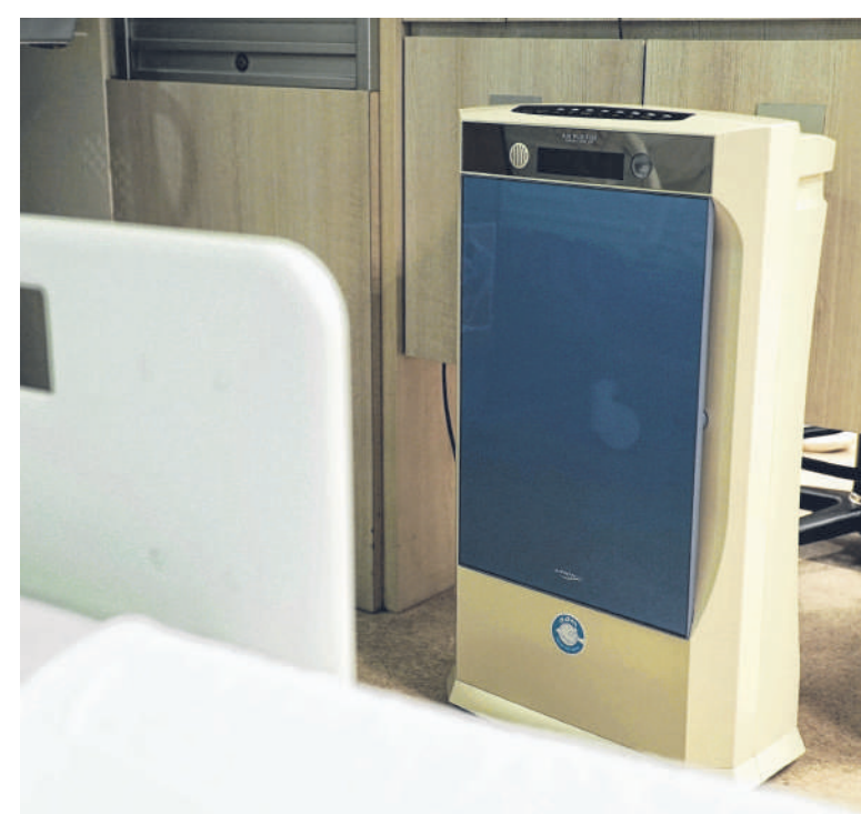
Each cubicle has a Hepa filter, which helps to remove airborne particles such as dust, mould and bacteria. ST PHOTO: MUHAMMAD AZIM AZMAN
