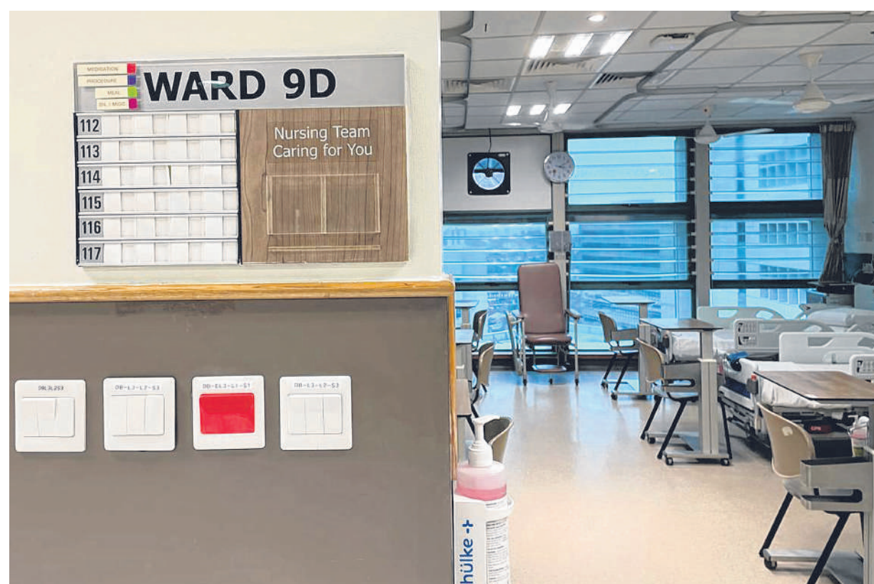
Ward 9D, which was the epicentre of Tan Tock Seng Hospital's Covid-19 outbreak, is reopening today. For better ventilation and air purification, the hospital has installed exhaust fans (one can be seen set into a window panel in the background) and portable high-efficiency particulate air (Hepa) filters in the C-class ward. ST PHOTO: CHERYL TAN
