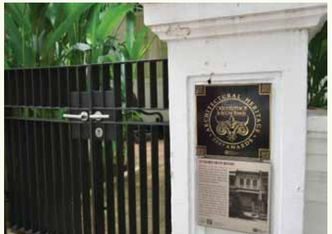
» 13 Martaban Road is a restored pre-war terrace house used as a dormitory for orderlies from Tan Tock Seng Hospital. Martaban was the old name for Mottama, a town located in the Mon State, Myanmar.
