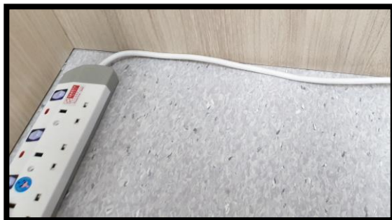
Taping of wire cords to the side of the floor.
