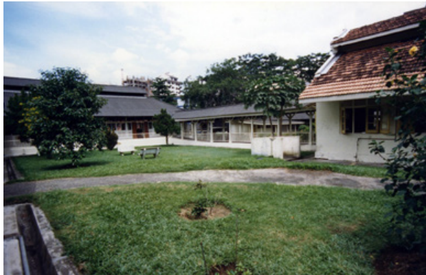
► Ward 60, Central Treatment and Kitchen Block
